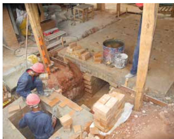
Construction of the new kiln
