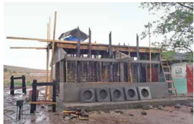
Construction of the new kitchen..
