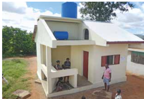
A new building for the school kitchen at Bel Avenir
