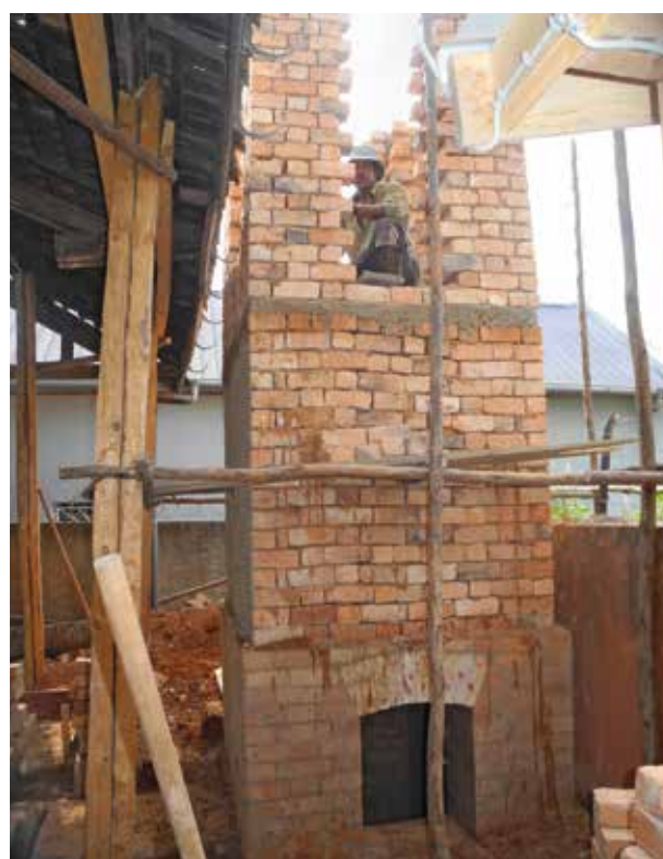
The chimney for the new kiln is almost finished.
