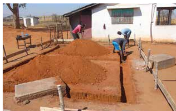
Construction starts on a new school kitchen at Ecole des Saphirs.
